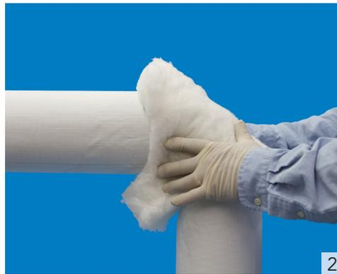
Place pre-cut Proto insert(s) around the fitting, positioning the insert on the inside radius of the elbow. In some cases, the insert can be secured and held in place with Proto PVC tape or filament tape.
