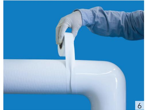
For an attractive finish, apply Proto's PVC tape around the circumference of the butt joints.
