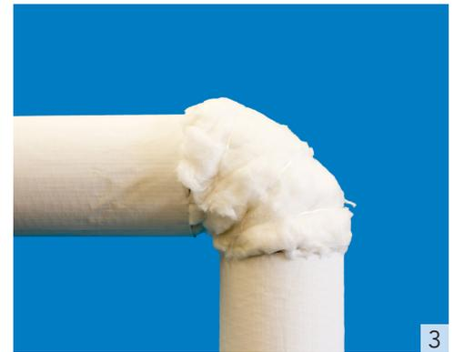
The edge of the Proto insert should be butted against the end of the pipe covering. Tuck and fold the insulation so it covers all bare surfaces. Care should be taken to not over-compress the insert. The insert(s) should be the same thickness as the adjacent pipe insulation.
