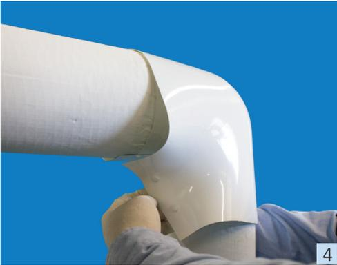
Insert stainless steel serrated tacks (2+ tacks per fitting) approximately 1/4" (6mm) from one of the lap edges of the fitting cover. For large or specialty fitting covers, use additional tacks to obtain a smooth, uniform fit. To assist with tack installation, form a small hole on one side of the fitting cover (using an awl or hole punch).
