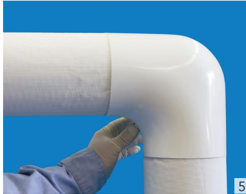
Once the fitting cover is in place, push the tack through the opposite side of the fitting cover. The serrated tack will firmly lock the fitting cover into place.
