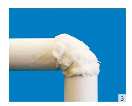
The edge of the Proto insert should be butted against the end of the pipe covering. Tuck and fold the insulation so it covers all bare surfaces. Care should be taken to not over-compress the insert. The insert(s) should be the same thickness as the adjacent pipe insulation.
