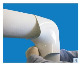
Insert stainless steel serrated tacks (2+ tacks per fitting) approximately ¼" (6mm) from one of the lap edges of the fitting cover. For large or specialty fitting covers, use additional tacks to obtain a smooth, uniform fit. To assist with tack installation, form a small hole on one side of the fitting cover (using an awl or hole punch).
