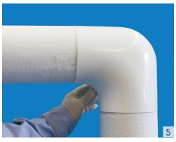
Once the fitting cover is in place, push the tack through the opposite side of the fitting cover. The serrated tack will firmly lock the fitting cover into place.
