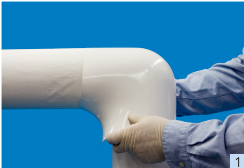
Position the Proto PVC fitting cover over the insulated fitting.
